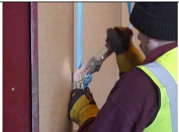
Photograph 4: Power grip when tightening the ratchet
